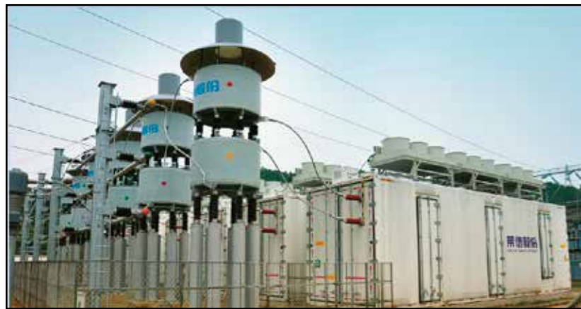
Figure 1: \pm 200\text{MVAR} , 500kV, outdoor containerised STATCOM system (Courtesy: Montnets Rongxin Technology Group Co., Ltd)
